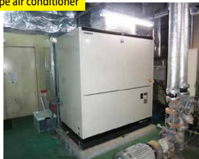
Gas heat-pump type air conditioner
