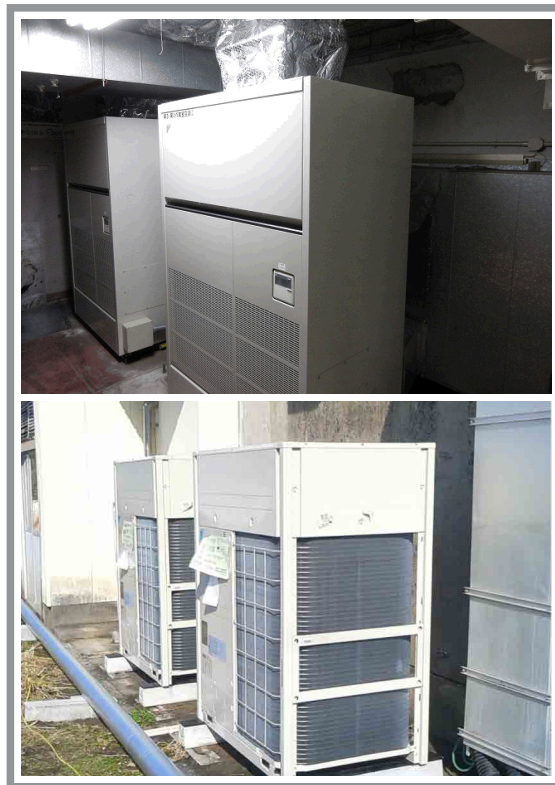
After replacement Air conditioners of electric package type
